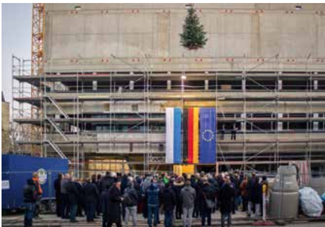
Topping-out ceremony in December 2016.
